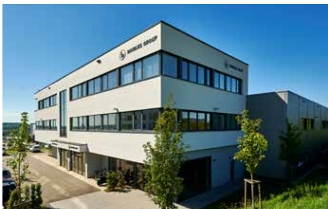
Baublies Headquarter in Renningen
